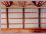
One 2 x 8 **Pressure Treated Bottom Board** Add to structural strength - and assure
